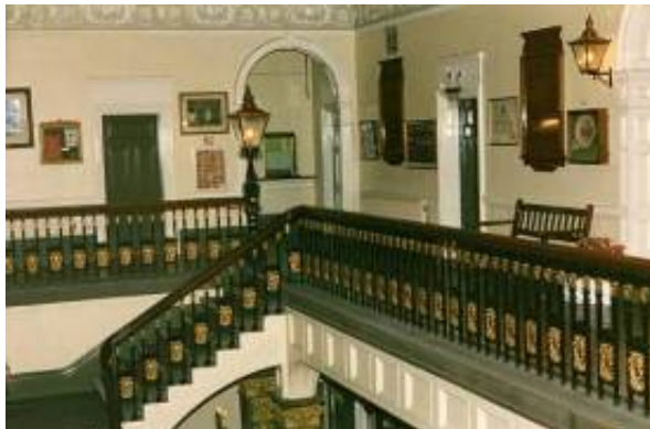
Central Stairwell, condition 1989
