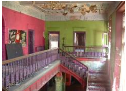
Central Stairwell, current condition
