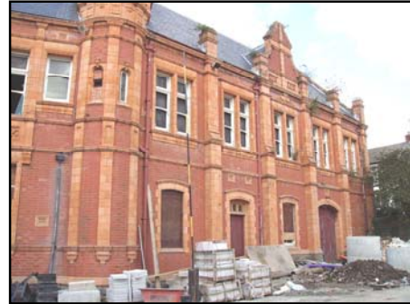
South Elevation (Car Parking Area)
