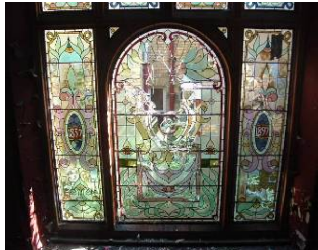
Stained Glass Window, central stairwell in current condition
