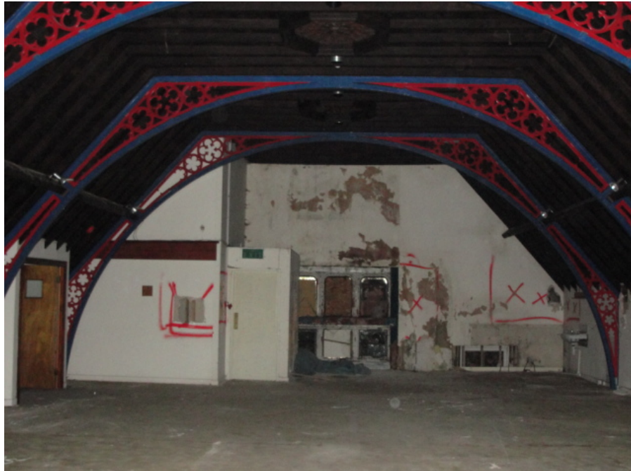
Second floor offices.
