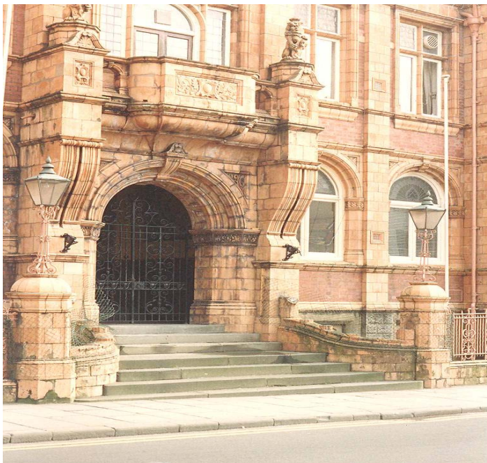
Town Hall 1989 –note windows
