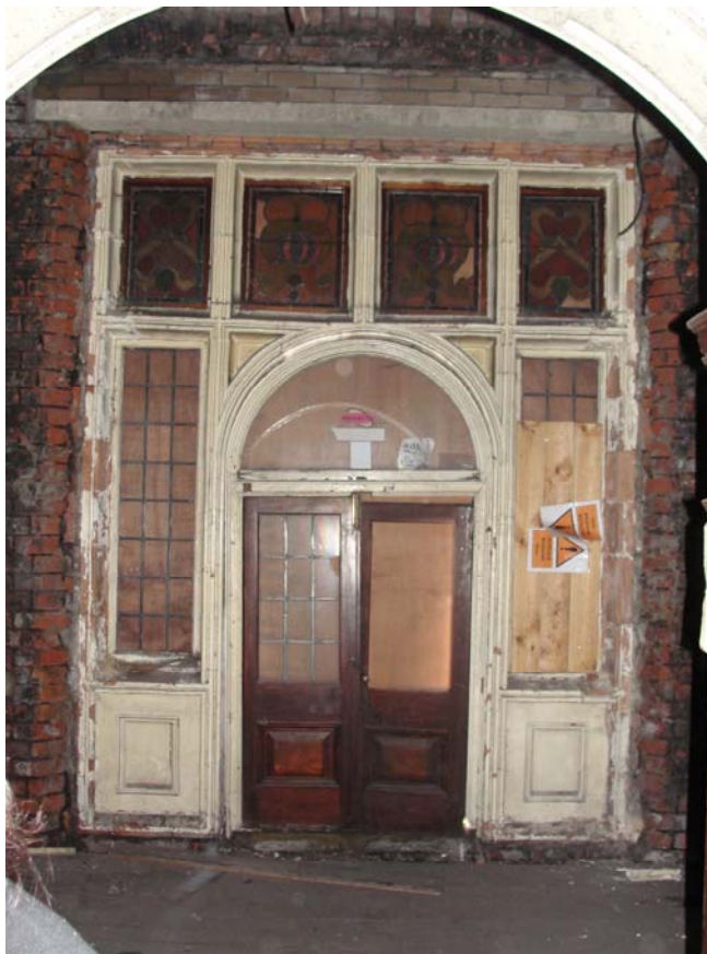
The Majors Office with Balcony windows.
