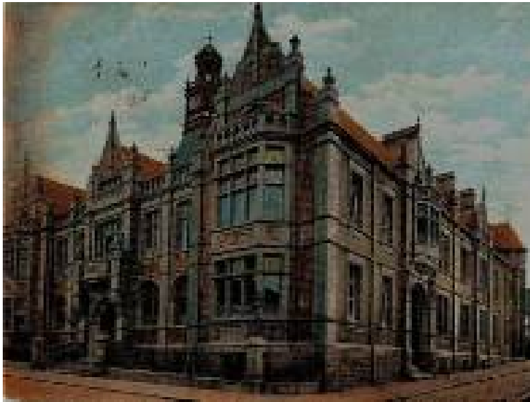
Town Hall 1899 – note windows
