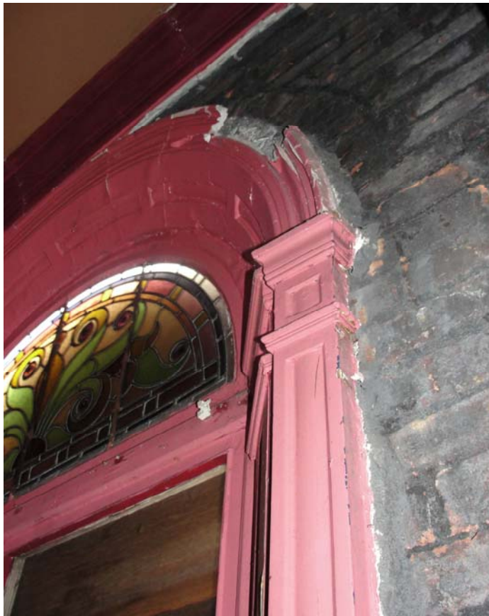
Front elevation windows showing plaster architraves.
